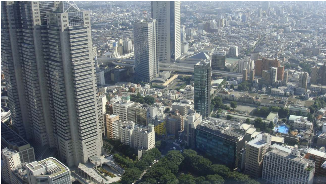
1 - View from the Metropolitan Building in Nishi-Shinjuku (Hotel Park Hyatt and EA Office)
